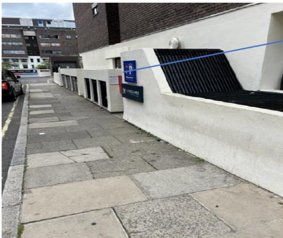
Harley Street Underground Car Park - PICTURES
